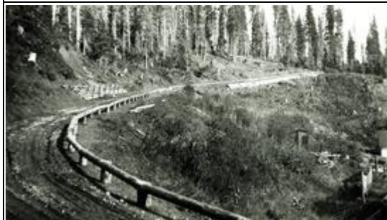
Young Men's Forestry Training Program (YMFTP) crew erosion control work and railing install on Aleza Lake road 1936
