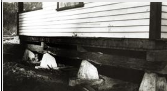
New sills and concrete footings installed under existing Aleza Lake buildings 1936
