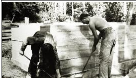
Removing forms from concrete reservoir 1936
